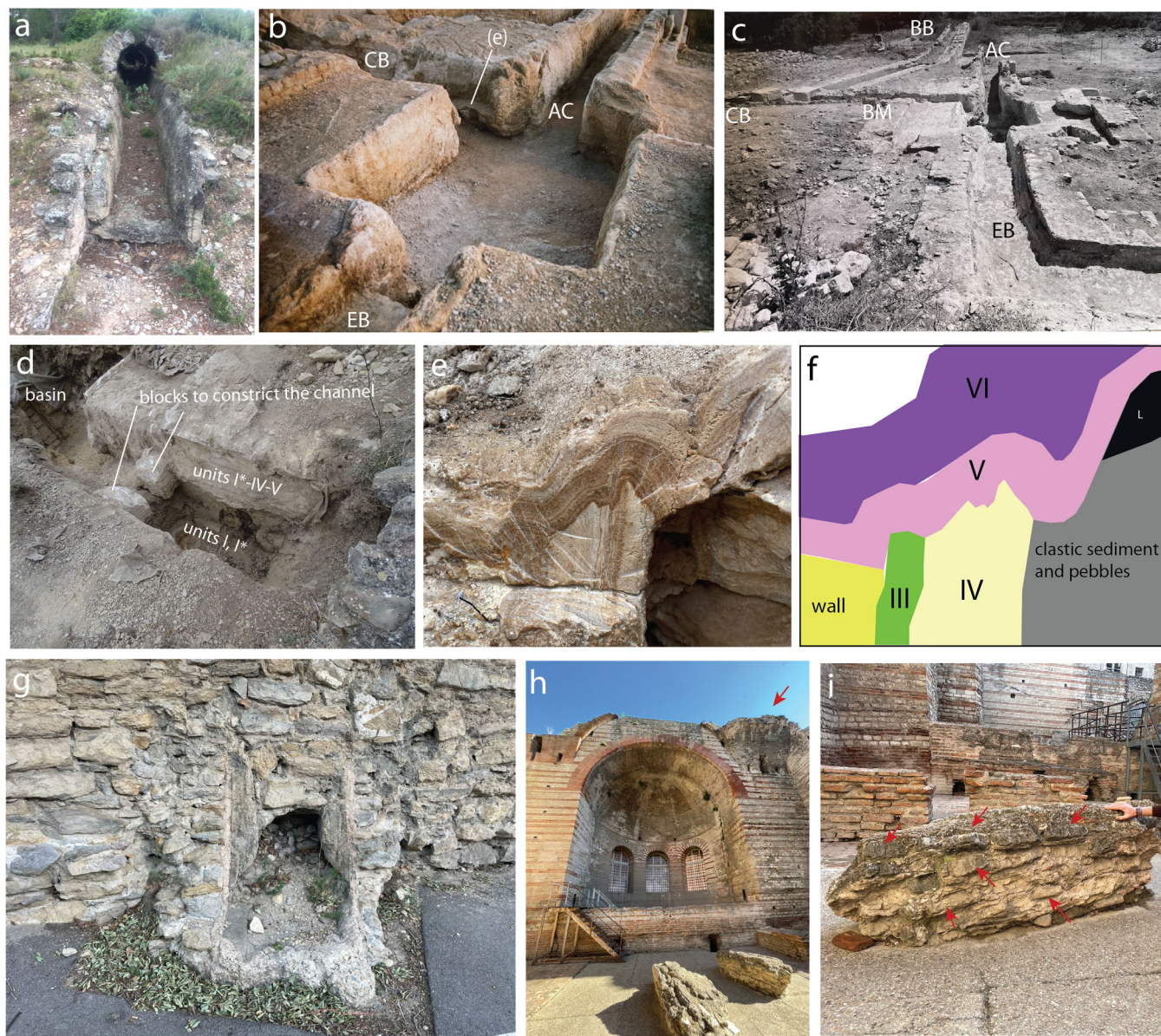
FIGURE 3 | Field observations of the Arles water structures. (a) Typical masonry channel section of the Eygalières branch, at the sampling site of AR09. (b) The Bassin des Arcs, looking south. (c) The Bassin des Arcs showing the feeding and outgoing aqueducts, looking south. (d) View of the 'bras mort', looking north. Clastic sediments were removed, exposing the bottom deposits of unit I and I*, and side deposits of units I*, IV and V. (e) Unconformity at the entry of the Caparon branch into the Bassin des Arcs, looking south, location given in (b). (f) Interpretive drawing of (e). An angular unconformity of unit V covers the partly breached wall that blocked the Caparon branch, and the sediments of units III and IV. (g) Arles city conduit close to where it enters the city of Arelate , at the sampling site of AR08. (h) Caldarium of the 'Baths of Constantine', Arles. Aqueduct carbonate fragments were used in the concrete of the vault of the caldarium, arrowed. (i) Masonry block fallen from the roof of the caldarium, consisting mostly of fragments of aqueduct carbonate embedded in mortar, arrowed. Sample ARC1 was sampled from this block. Photos (b) and (c) Philippe Leveau; other photos Cees Passchier. AC, Arles city conduit; BB, Barbegal branch; BM, bras mort; CB, Caparon branch; EB, Eygalières branch.
