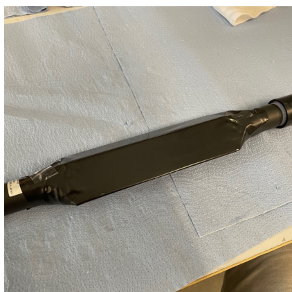
(a) Foil seam covered with sealing tape.
