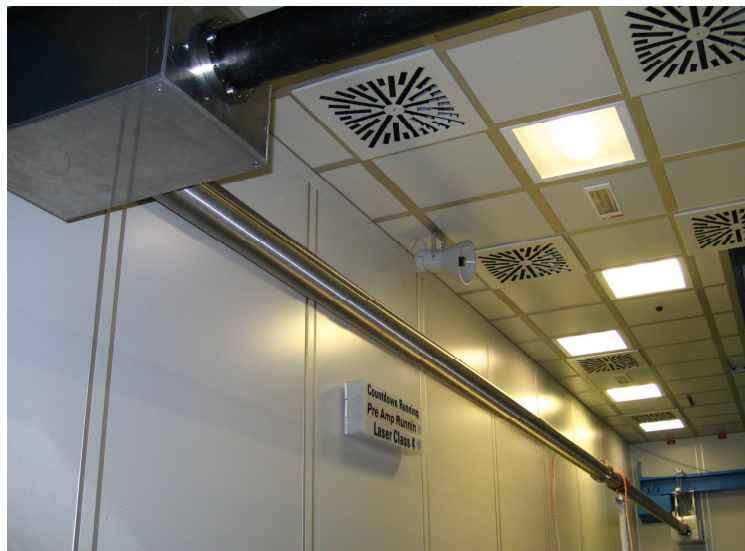
Figure 50: Transport beamline across the PHELIX laserbay towards the reinjection channel.
