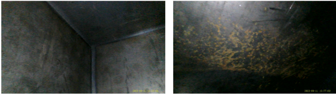
Figure 6.25: Endoscopic photos showing selected areas of the inner detector walls with and without oxidation.
