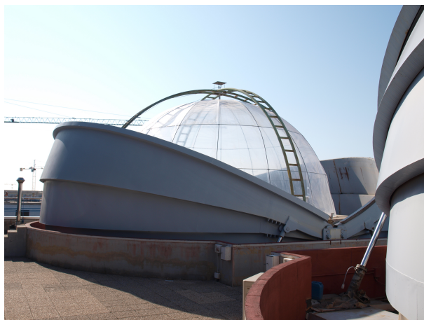
Fig. 5.1: EUPHORE chamber in Valencia while opening the roof to start the experiments.
