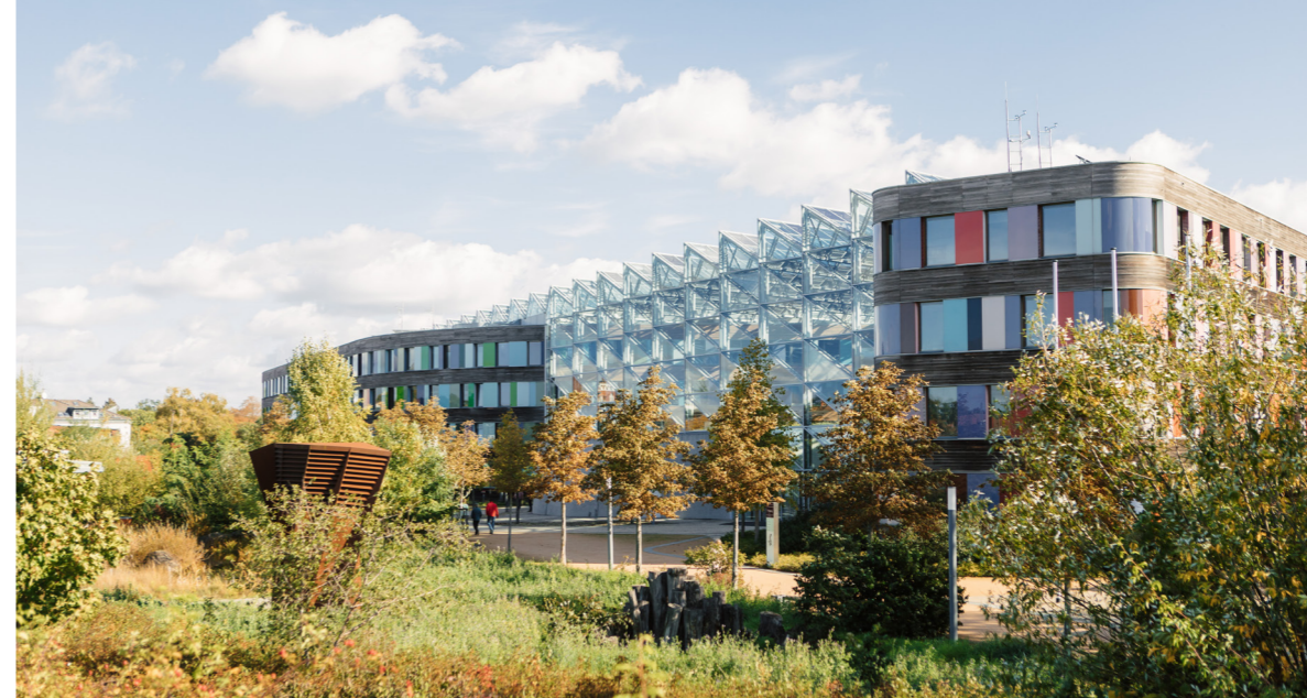
Fig. 21: The German Environment Agency in Dessau. By Sauerbruch Hutton Berlin. 2005. Photo: Sebastian Köhler, Stadtmarketinggesellschaft Dessau-Roßlau mbH
