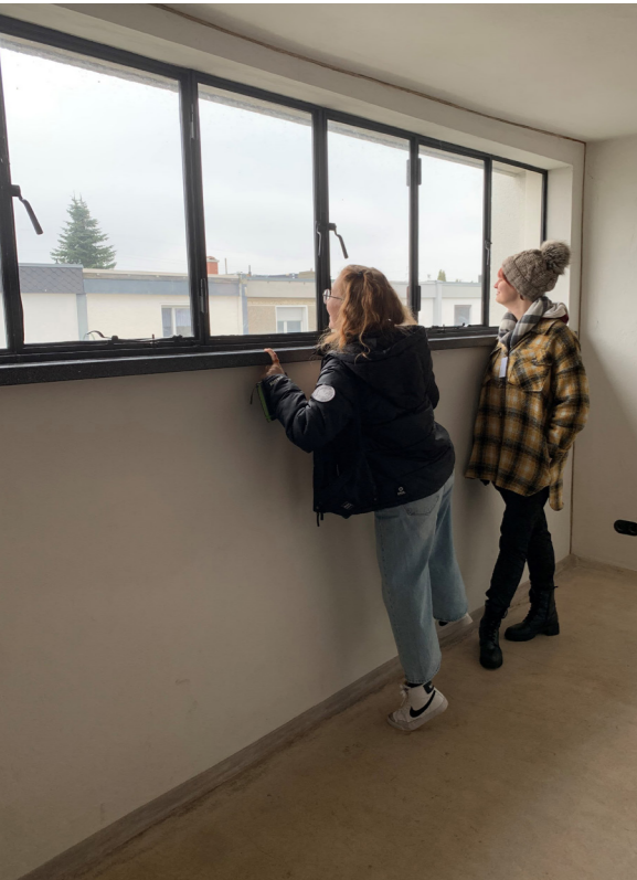
Fig 12. Upper floor reconstructed Haus Anton: the windows are installed at their original height, March 2023, Photo: Regina Stephan
