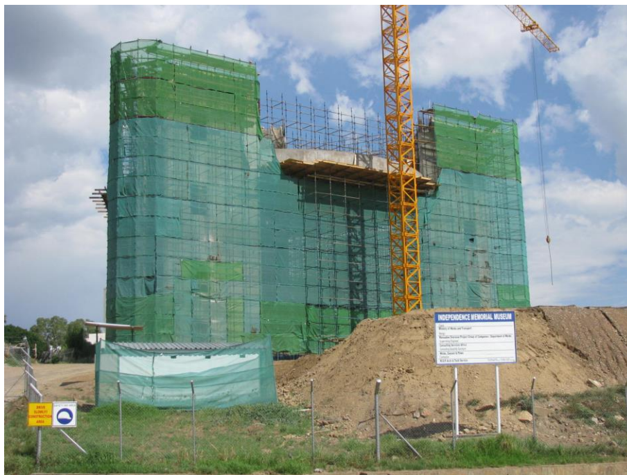
Fig. 29: The Independence Memorial Museum under construction, March 2010. Photo: Godwin Kornes (2010).
