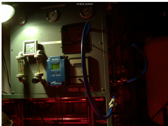
Figure 3.35: The most important aspects of the water system and HV monitoring systems are shown. The left plot shows the camera picture of the water filtration system that is regularly inspected with respect to the water flow rate, water temperature and water conductivity. The right plot shows the summary section of the HV monitoring website.
