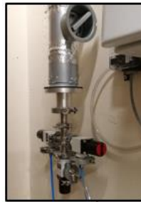
Figure 11 : ventilation pipe to exhaust gas
