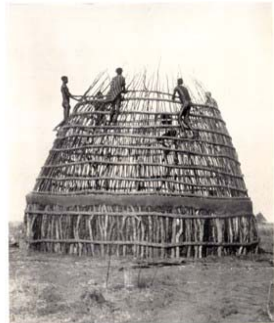
Building a cattle byre (Eastern Jikany)
