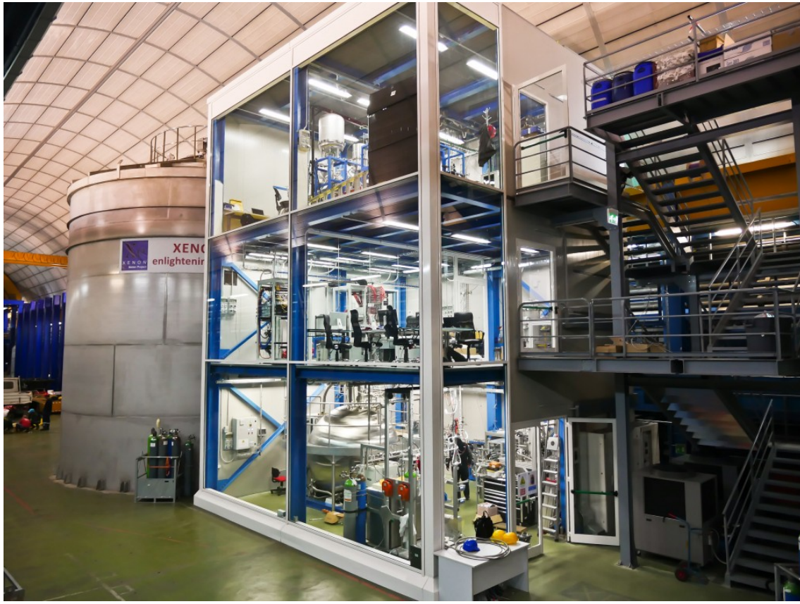
Figure 2.8.: Picture of the the whole XENON1T experiment, situated in Hall B of the Laboratori Nazionali del Gran Sasso (LNGS) in Italy. On the left hand side the water tank is visible which sits right next to the three story service building with its glass walls. The ground floor holds the xenon storage system ReStoX and the purification column [15]. In the first floor are the DAQ system and slow control together with an office. The upper floor is home to the gas system [12].
