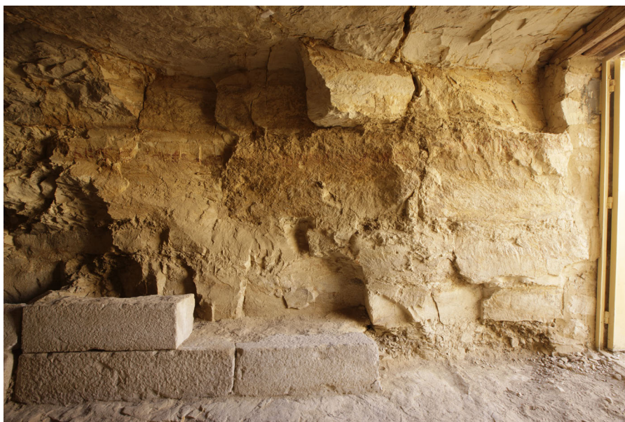
Fig. 9: Inscriptions in red paint on the western wall of Shepesuptah's rock-cut chapel, which was originally covered with limestone casing (photograph Czech Institute of Egyptology FF UK, Martin Frouz).
