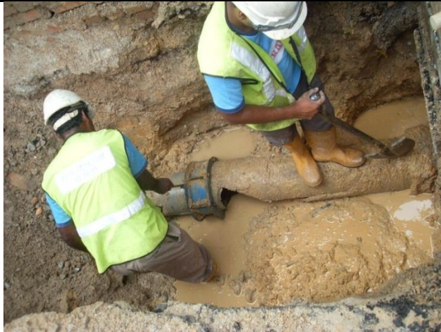
Joint failure
