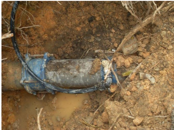
Replacement of AC pipe with PVC
