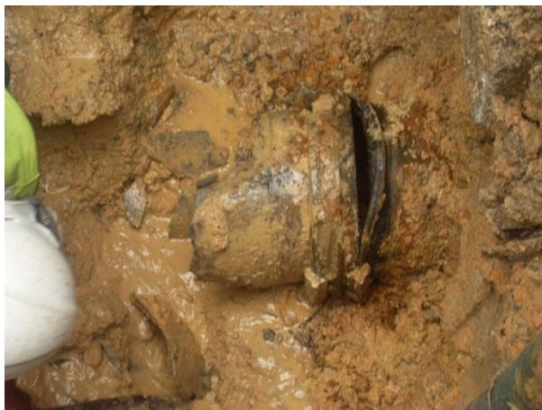
Joint failure
