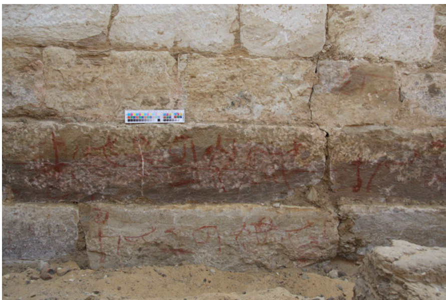
Fig. 8: Builders' inscriptions and a levelling line on the western wall of Inpunefer's tomb (photograph Czech Institute of Egyptology FF UK, Hana Vymazalová).
