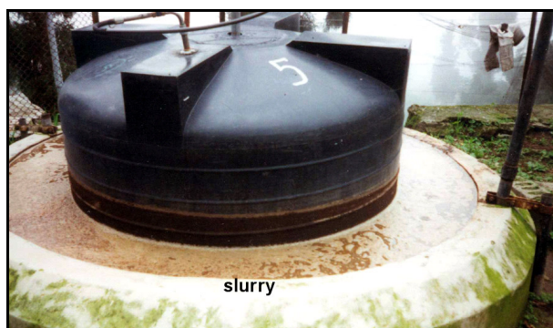
Photo 5.44: Floating biogas tank and slurry, a methane gas by-product, Darjeeling District (Photo by SHILPI SAXENA, 2002)
