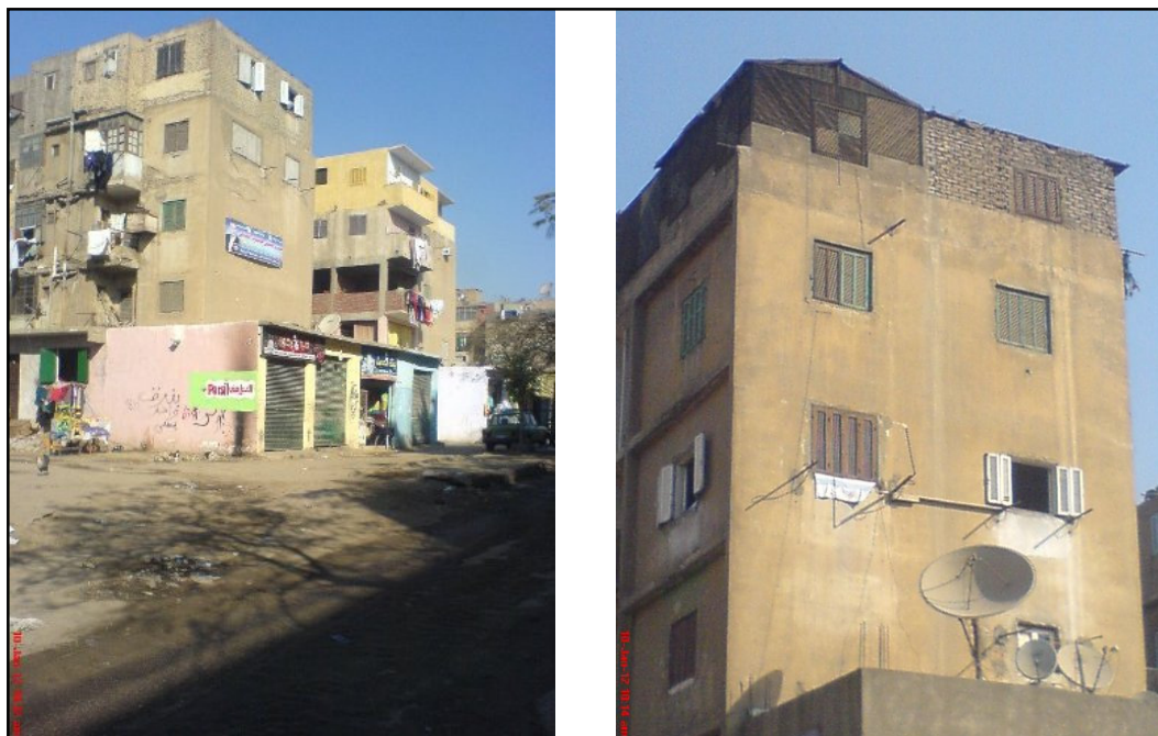
Fig. 46: Informal building activities in Ain el-Sira public housing
