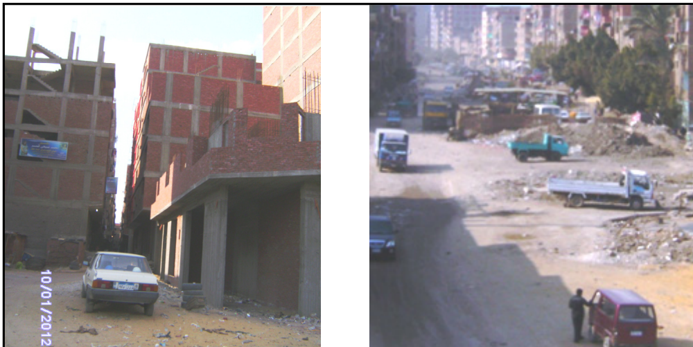
Fig. 42: Examples of the width and conditions of streets in EI-Marg el-Qibliya. The left picture shows a disproportionate street width with regard to the building heights, and the right picture shows lack of paving and accumulation of sewage in the main streets. Source: Author's photo.
