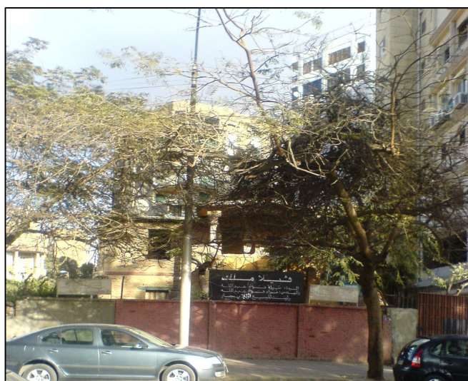
Fig. 52: Old villa beside high rising residential buildings in El-Nozha
