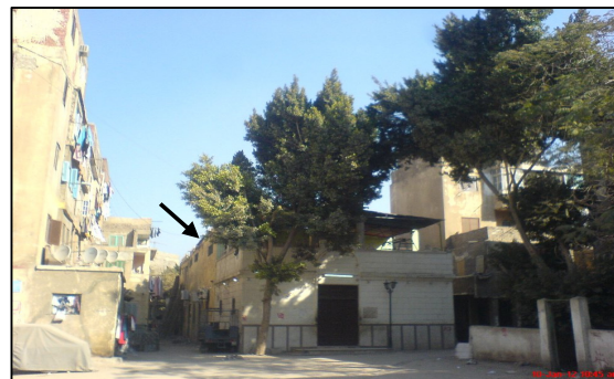
Fig. 69: Indigenous mosque in the spaces between the building blocks in the governmental housing of Ain el-Sira
