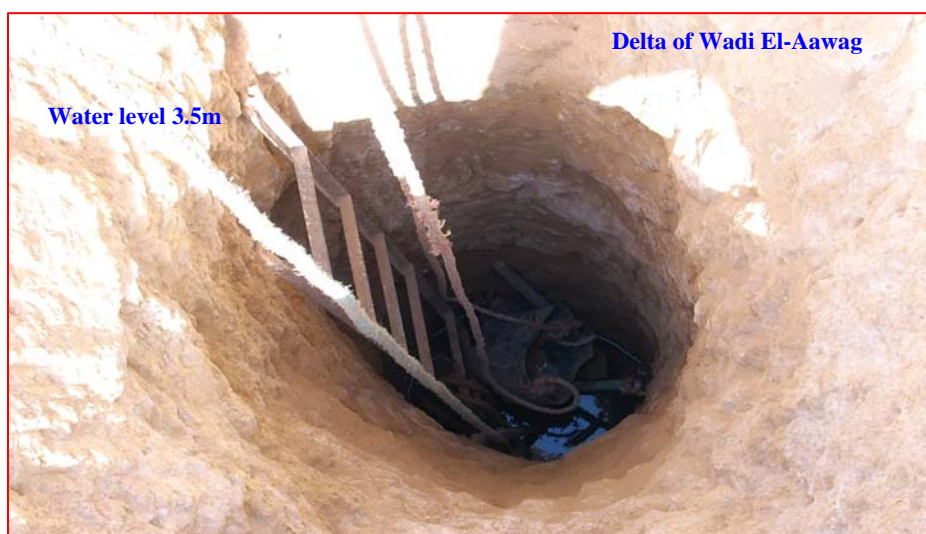
Photo (5-3) Water level is 3.5m deep in a well of the delta of Wadi El-Aawag north of El-Tur.
