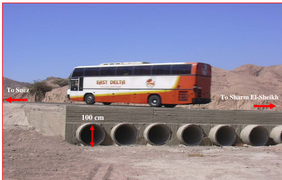
Photo (5-6) Culverts of the highway Suez- Sharm El-Sheikh
