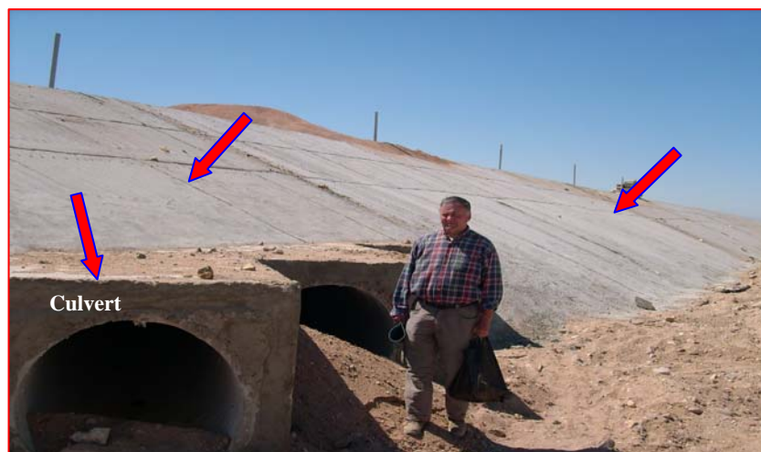
Photo (5-9) Construction of diversion the main channel of Wadi Firan
