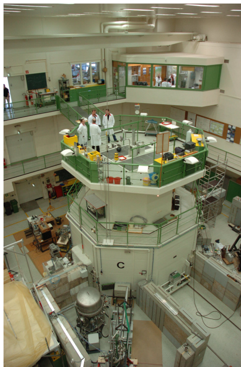
Fig. 3.3. The TRIGA Mark II – Reactor at the Institute of Nuclear Chemistry, University of Mainz ( kernchemie.uni-mainz.de/234.php ).
