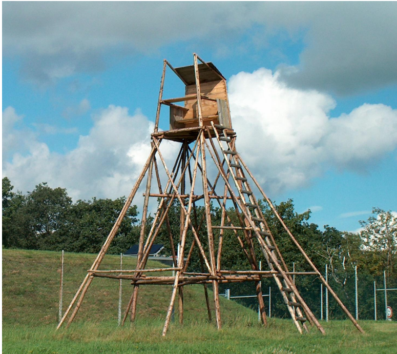
Figure 2. One of 10 wooden towers built for the bat monitoring in the SAC 'Ahringsbachtal', used to to maximise the perception range of the transmitted signals.
