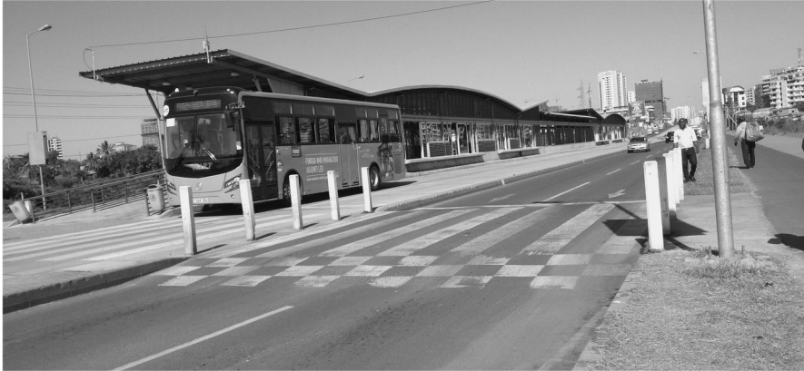
Fig. 3 Pedestrian crossing with speed bump at a station. Author's photo (2016)
